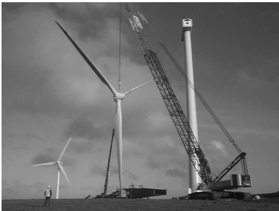
Figure 5 Construction at Woolnorth Wind Farm, Tasmania.
