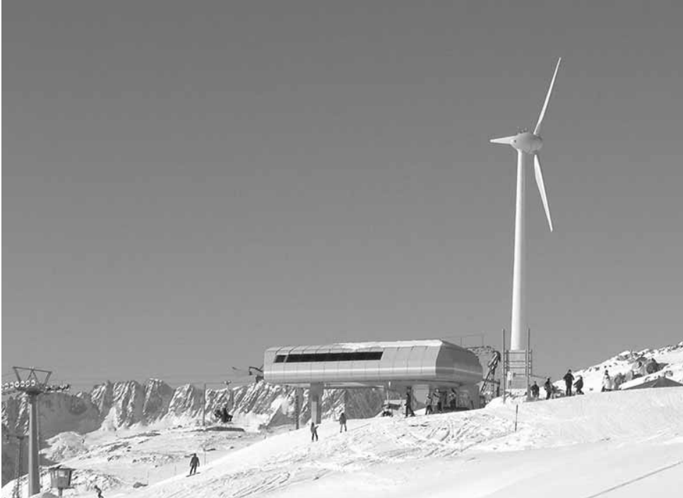
Figure 2 Wind turbine at a walking distance from a ski lift in Gütsch. Turbine is equipped with a de-icing system. Photo: ENCO AG, Switzerland.
