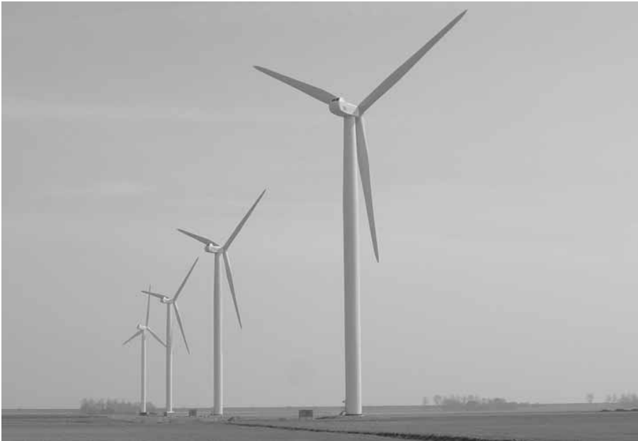
Figure 3 Nordex 2.5-MW turbines at ECN test site Wieringerwerf. Photo courtesy of Jos Beurskens.
