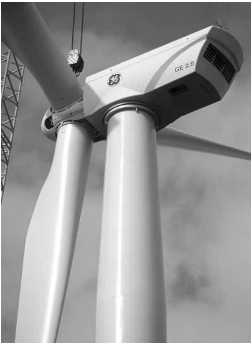
Figure 4 Erection of the GE Wind 2.5-MW turbine at the ECN test site. Photo courtesy of General Electric Wind.
