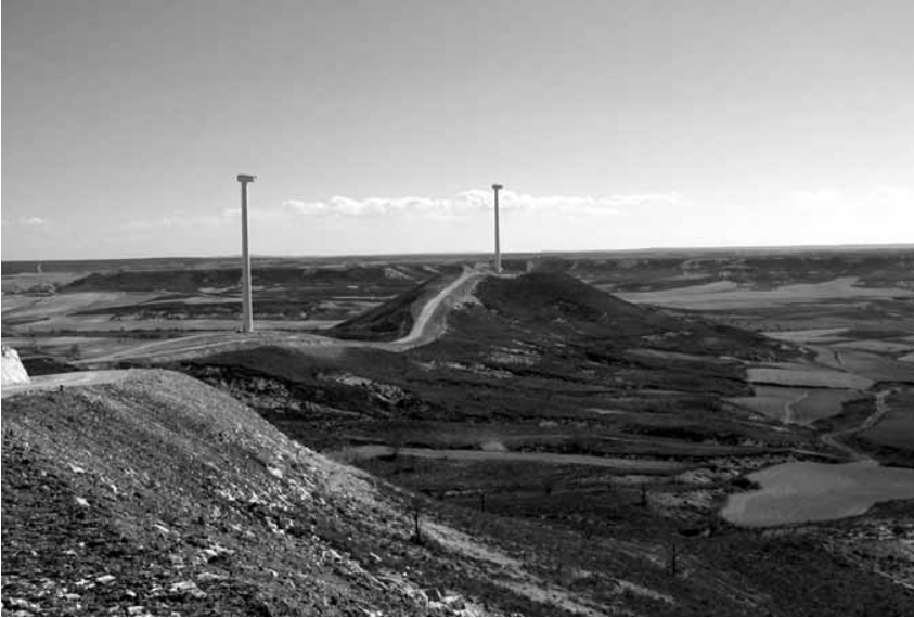
Figure 6 Wind farm under construction in Castilla-Leon.
