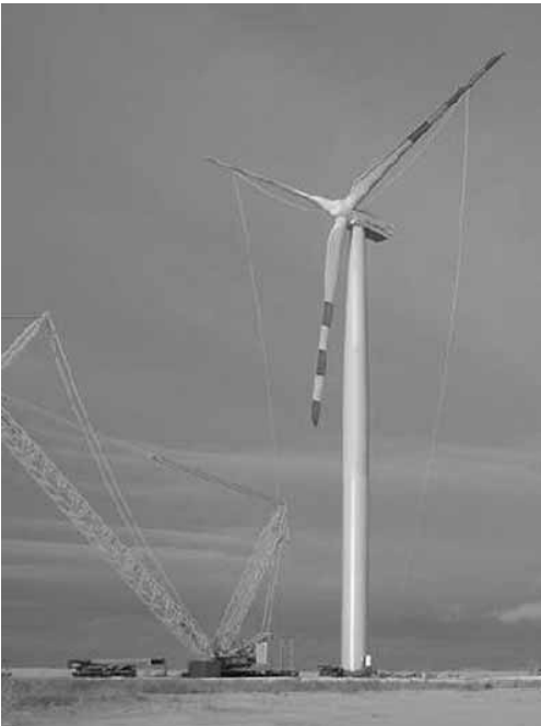
Figure 4 Erection of 3-MW pilot turbine by WinWinD, November 2004, Oulu, Finland.
