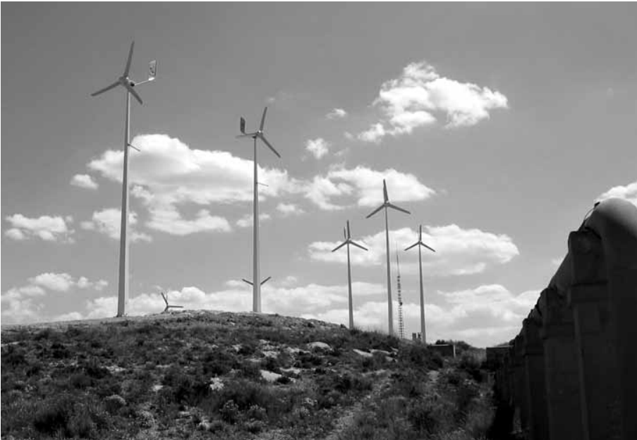
Figure 8 Wind farm with small wind turbines (5kW grid connected).
