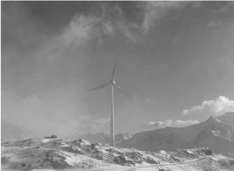
Figure 3 Enercon E-40, operating on Mt. Gütsch, 2,340 m above sea level.
