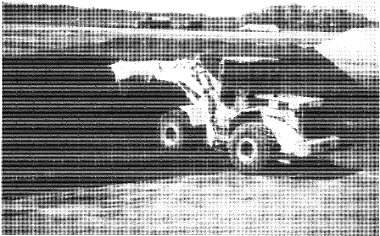
Figure 7.6 Stockpiled Asphalt Emulsion-RAP Maintenance Mix
