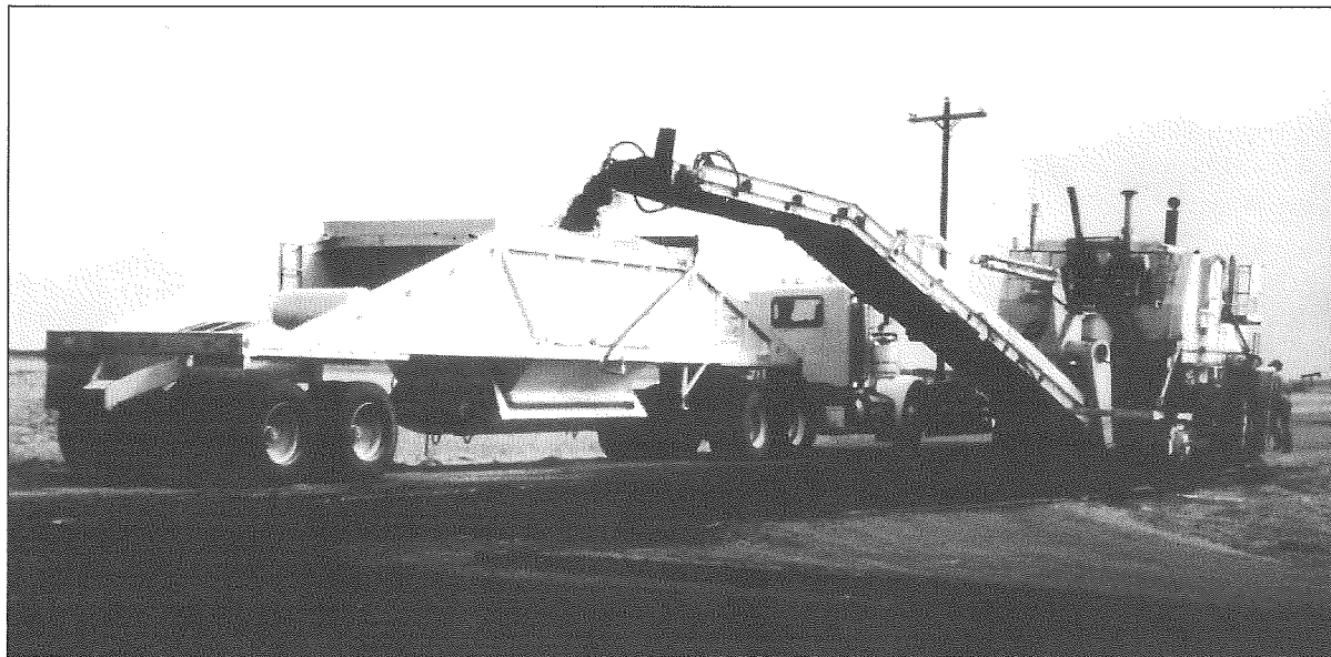
Figure 9.3 Cold Planing/Milling Machine Removing Asphalt Pavement
