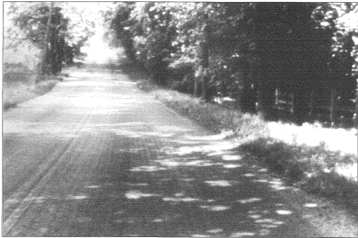
Figure 6.15 Longitudinal Streaking
