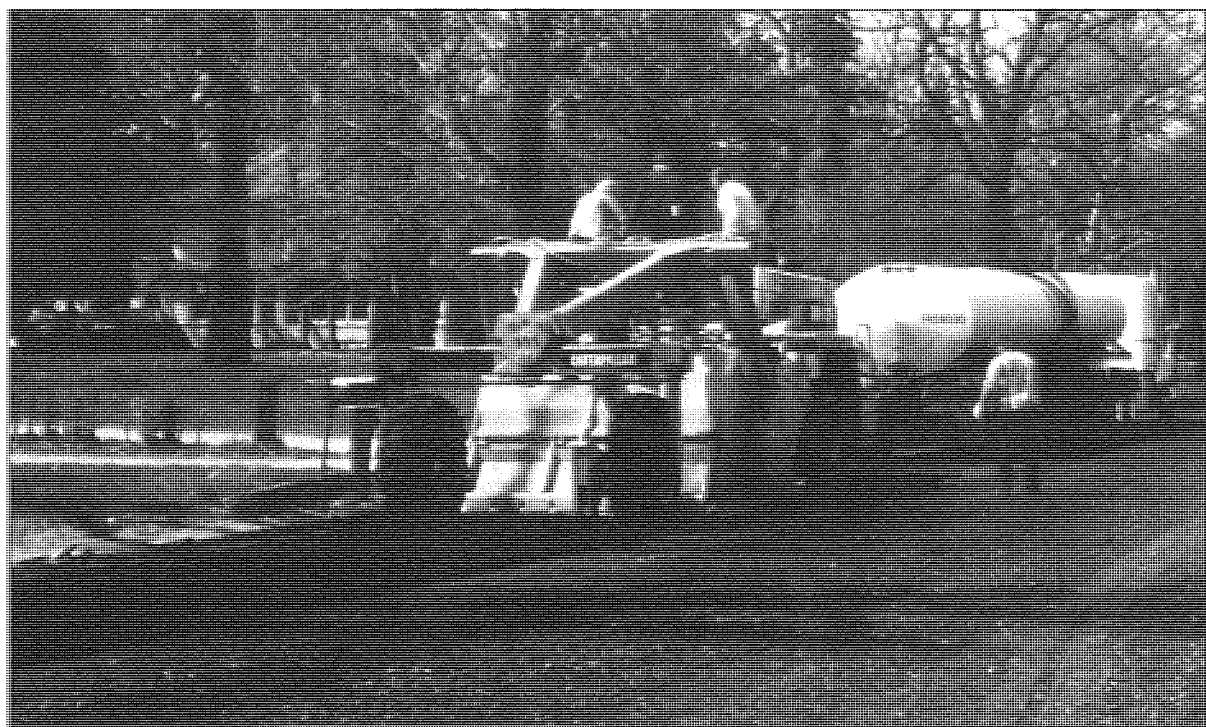
Figure 9.6 Asphalt Pavement Reclaiming Machine Adding Asphalt Emulsion
