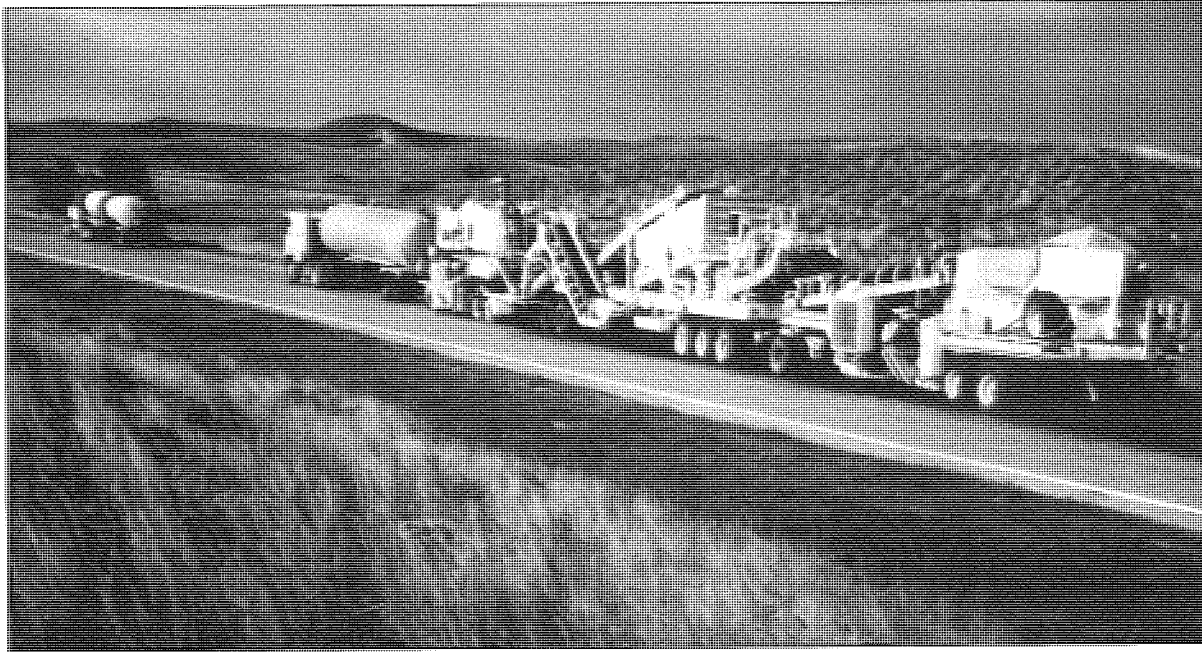
Figure 9.5 Multiple Unit or "Train" for Cold In-Place Recycling
