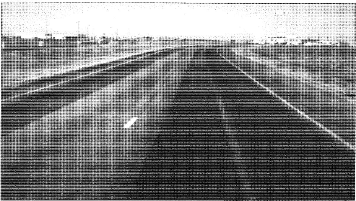
Figure 6.16 Bleeding Asphalt
