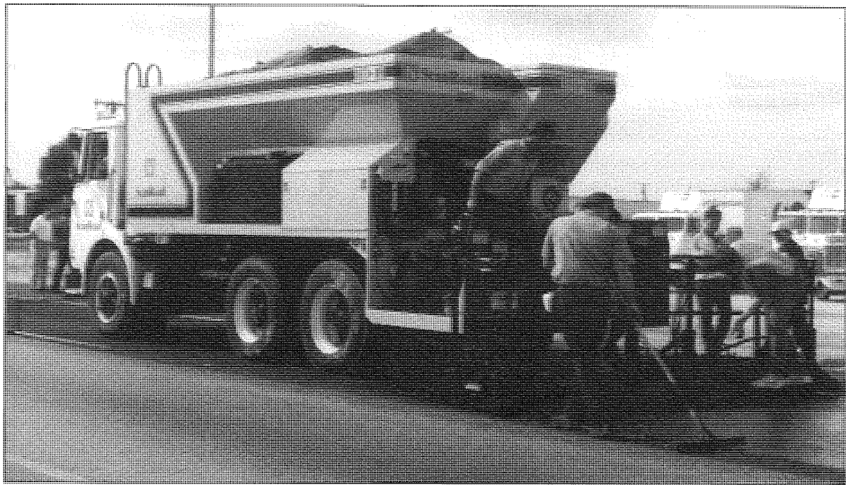
Figure 6.2 Slurry Seal Equipment
